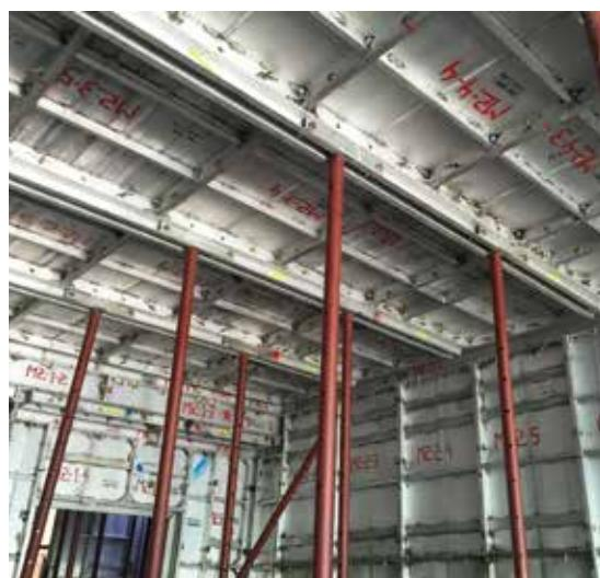
▲ Build smart - Doka Aluminum Formwork System produced by MFE allows highly cost-effective forming achieved by an adaptive and logical system concept
