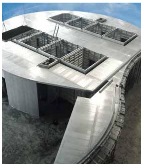
▲ Exact adaption to project specific requirements eliminates adjustment work on site and speeds up forming time
